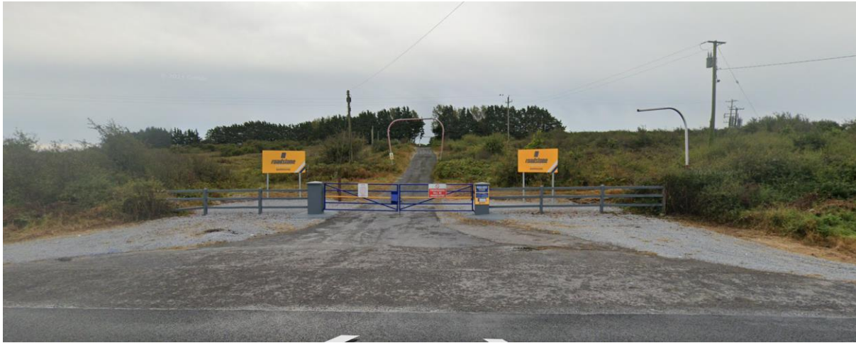
Figure 4-3 OCGT site application area entrance along the N69.
